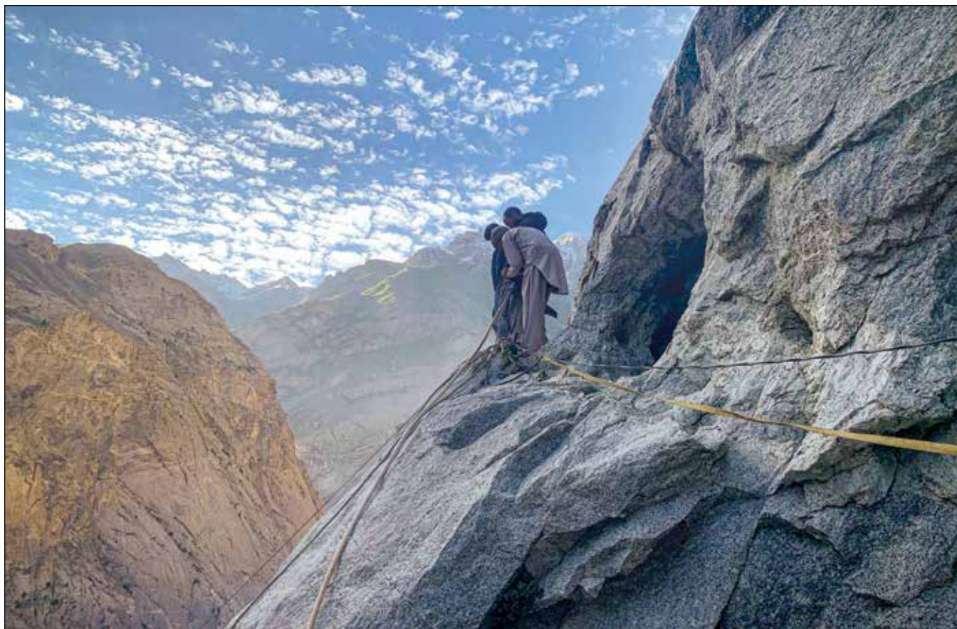
Figure 41 (above). Anchoring the cable near the mine portal.
