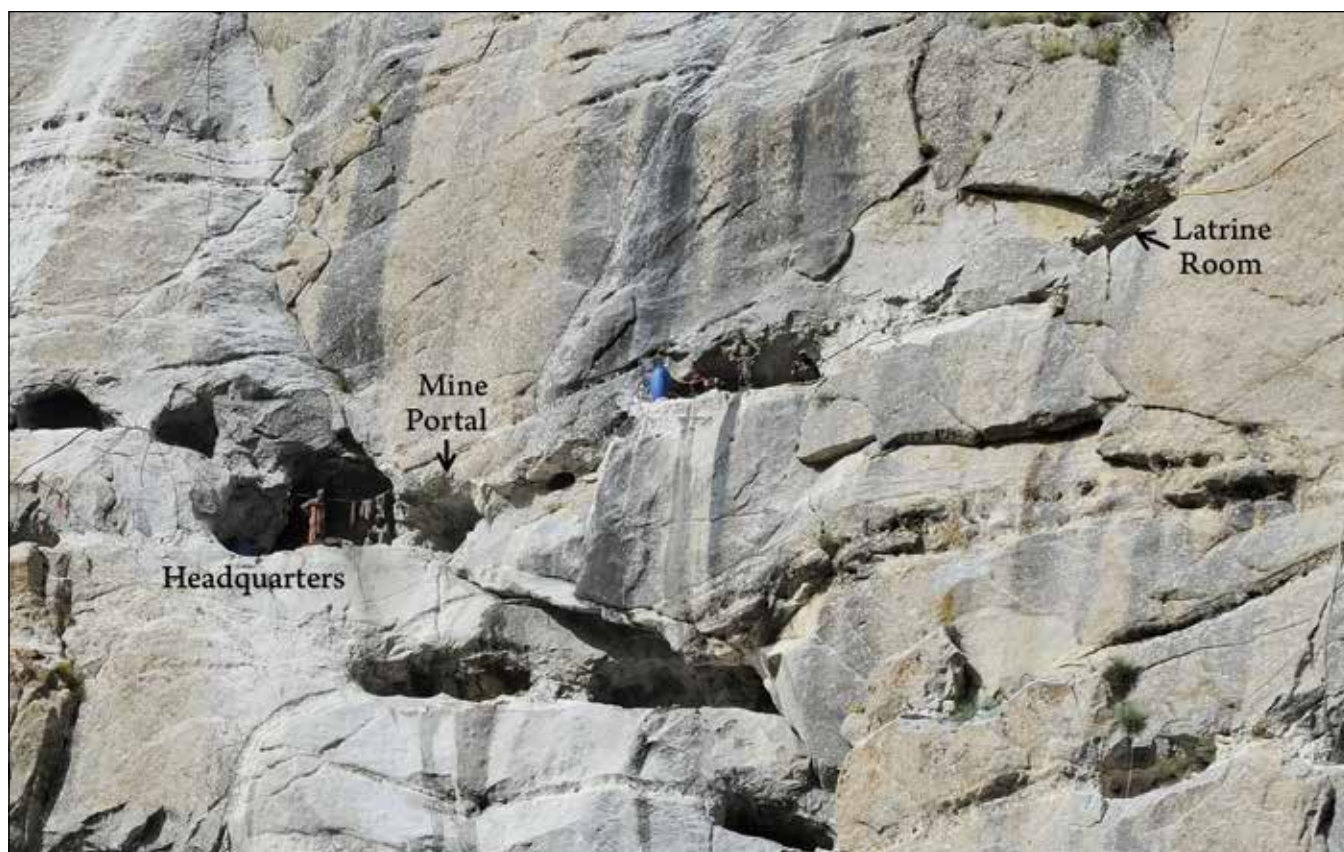
Figure 34. Locations of the “Headquarters” tunnel, the mine portal, and the cliff ledge leading to the latrine area. Note the cable strung as a hand-hold leading to the latrine. Fine Minerals International photo.
